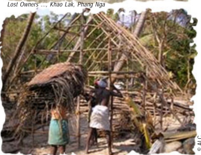
Building of temporary houses for those affected
